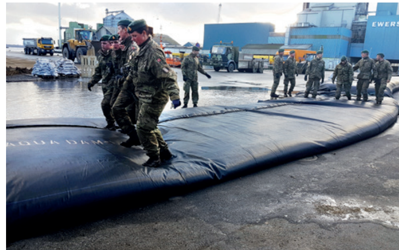
Rising water levels in Southern Jutland. IGR has been called in to help prevent flooding
